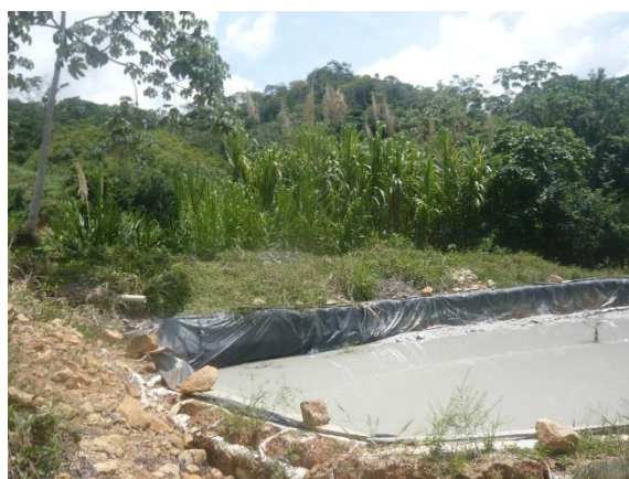
Figure 13. Pool with cyanide or mercury leachate waters. Source: r3 Environmental Technology Colombia SAS, 2016
